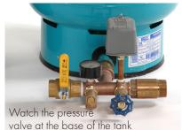
Ideally, it should take more than one minute of run time from the time it clicks on until the time it clicks off. In no event should it take less than 20 seconds. If it is less than 20 seconds, it indicates your tank may need to be replaced. If the cycle is somewhere around 50 to 10 seconds, it needs immediate attention or the pump will burn out.
