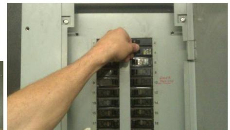
If you have an **electronic pump protection**, you will have to let it run through its time cycle, or reset it by snapping the circuit breaker off and then on again. It is set for a predetermined amount of time in the off cycle to allow the well to recover after it has been over pumped, thus tripping the shut off.
