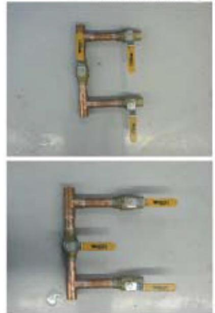
**PHOTOS:** The top photo shows how the shutoffs look when the water is off. The lower photo shows how the shutoffs look when the water is on.
